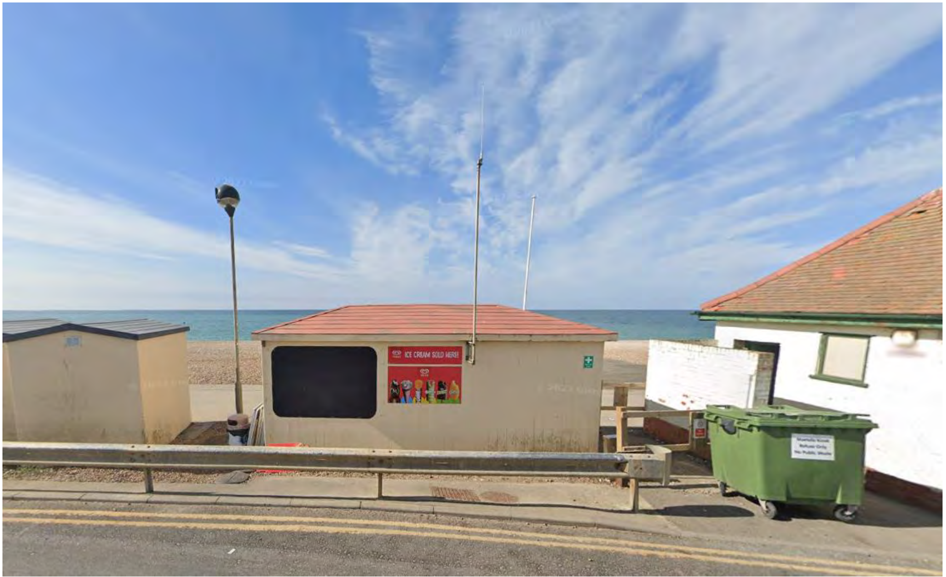
View SW of the Martello Kiosk, from The Esplanade
